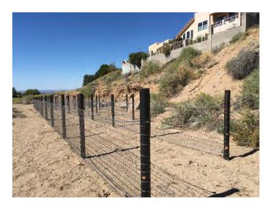
Erosion control system constructed by COA Hydrology in Bear Canyon West (Project 9)
